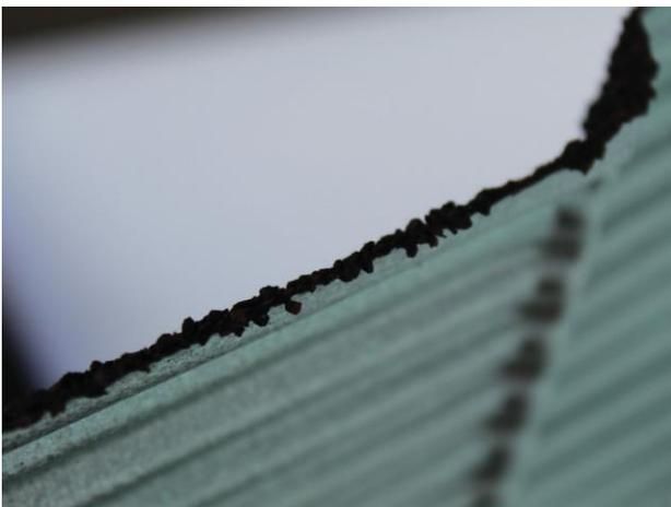
Stone granules at the edge of a tile, this may be removed during installation and handling. This chip may end up being washed down into the gutter.
