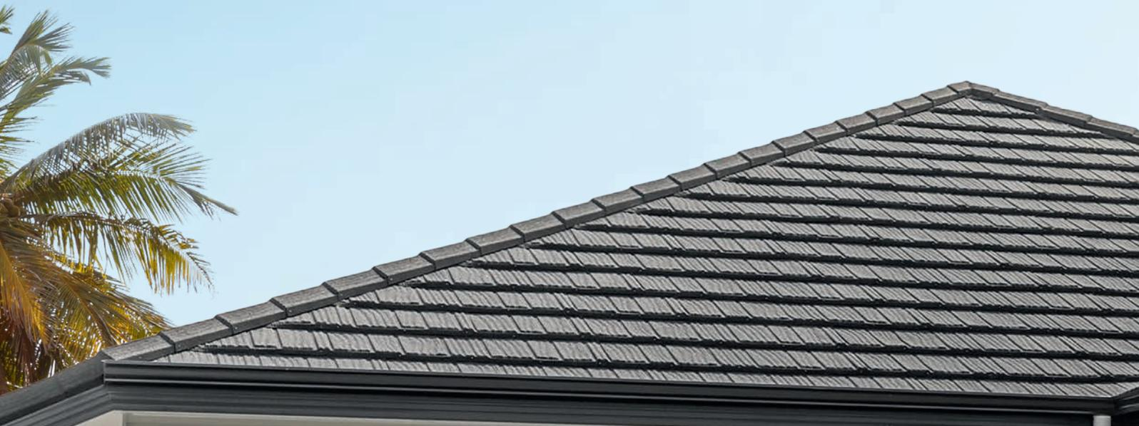
Because the interlocking panels are fixed horizontally, a Gerard roof is significantly more secure in high winds than vertically fixed roofs like concrete tiles or corrugated metal roofing.
