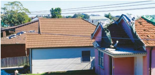
Sydney 1999: The Gerard roof in the centre remains intact; houses on either side with concrete and clay tiles sustain major hail damage.
