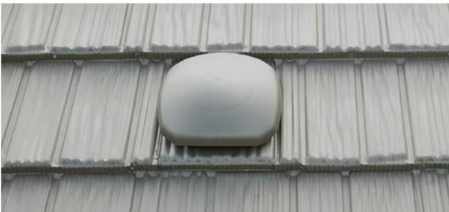
A low-profile port designed for extraction systems from kitchens, bathrooms and laundries. And with a large free vent area, it's also ideal for airflow and heat circulation in roof cavities.
