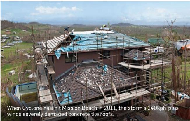
When Cyclone Yasi hit Mission Beach in 2011, the storm's 240kph-plus winds severely damaged concrete tile roofs.
