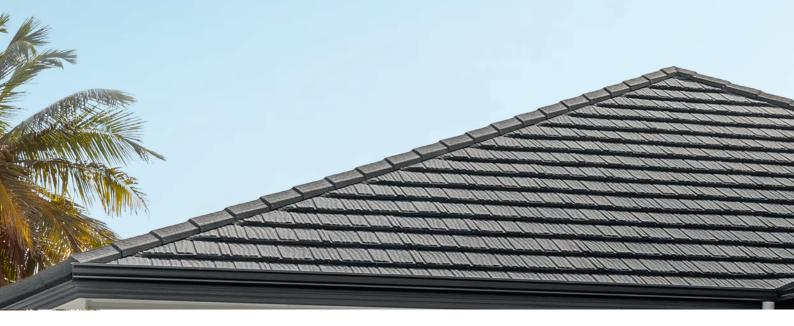
Because the interlocking panels are fixed horizontally, a Gerard roof is significantly more secure in high winds than vertically fixed roofs like concrete tiles or corrugated metal roofing.
