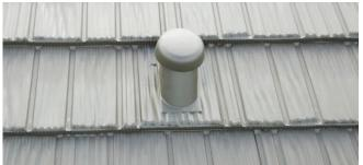
Primarily intended to vent sewage systems, this port can also be used for general air/moisture extraction from kitchens, bathrooms and laundries.
