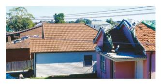
Sydney 1999: The Gerard roof in the centre remains intact; houses on either side with concrete and clay tiles sustain major hail damage.
